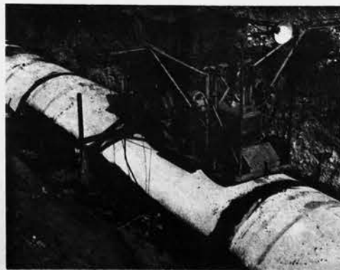
A special machine was developed to travel along the length of the water pipe, and press down sand covering surrounding it.
